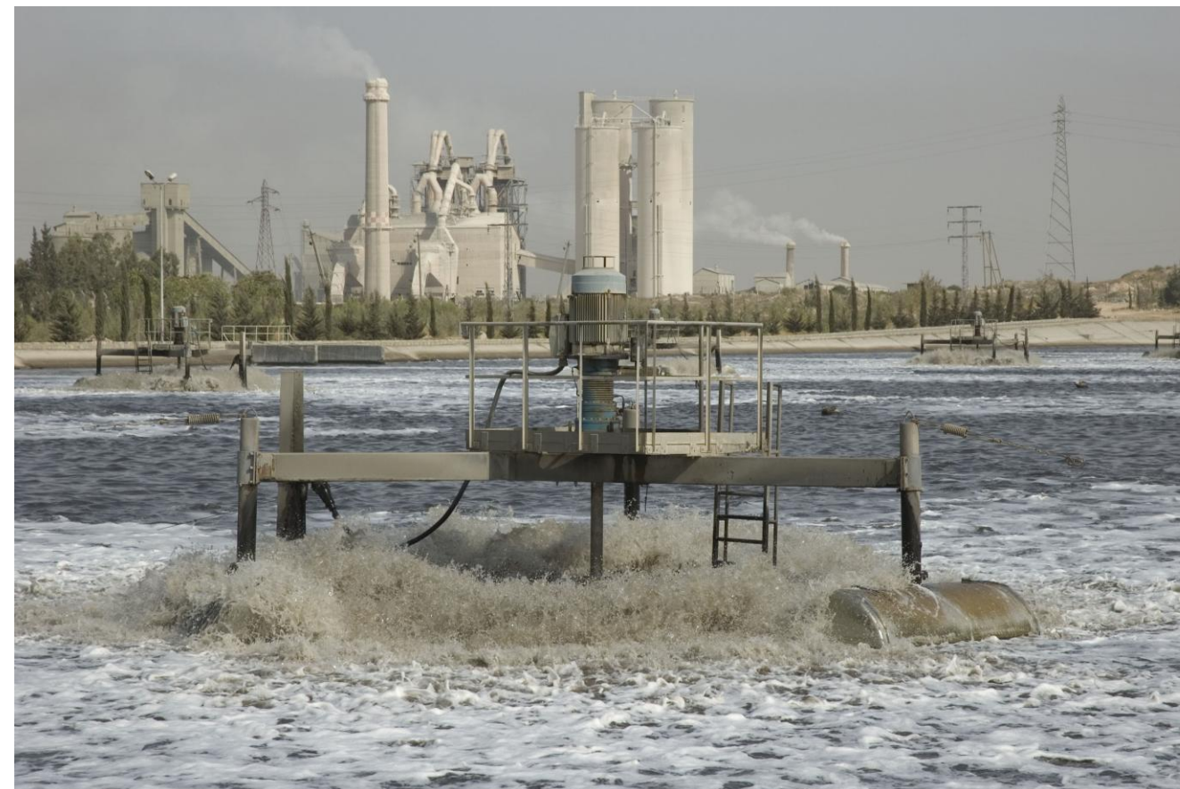
Energy neutral treatment plants
